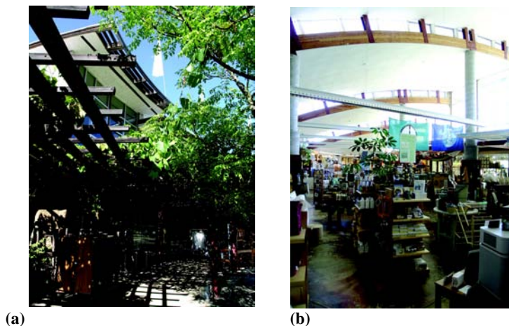
Figure 4-8. (a) The entry elevation of Real Goods Solar Living Center makes use of overhangs, a recycled-redwood trellis, and adjustable awnings. (b) The interior reveals its curving, stepped roof, east-facing clerestory windows, and light shelves that deliver natural light deeper into the interior without overheating or glare.
