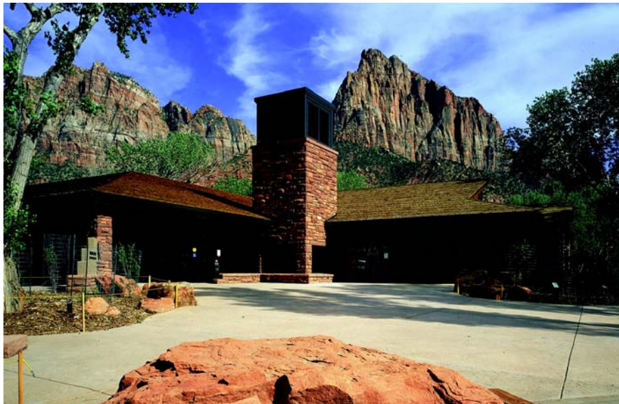
Figure 4-11. Zion National Park Visitor Center and Bookstore entryway showing the downdraft cooltowers and overhangs.
