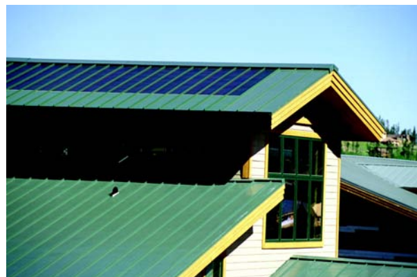
Figure 4-14. (a) Daylighting controls dim lights when there is enough natural light. (b) Solar panels on the roof and clerestory windows.
