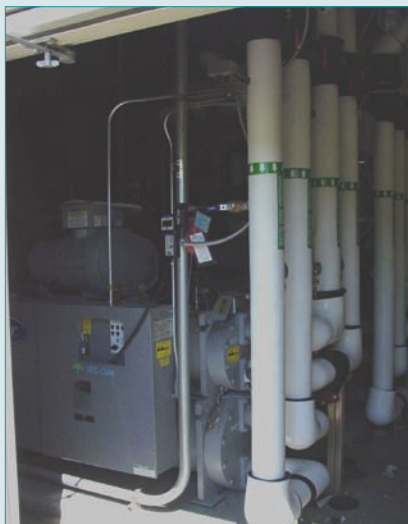
Figure S7.1. Water source heat pump.
