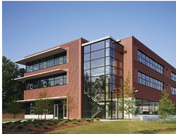
Figure 4.7. Building exterior with light shelves.
