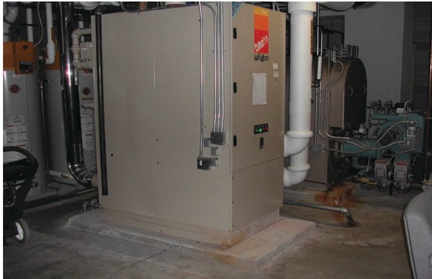
Figure 4.18. Pulse condensing boiler.
