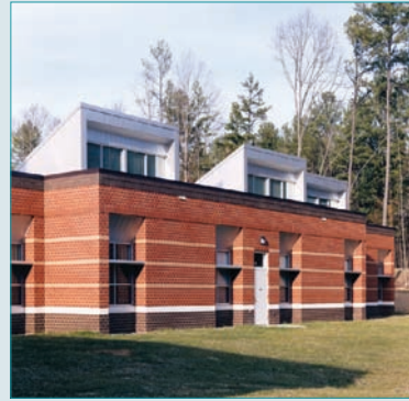
Figure S4.2 South-facing monitors.
