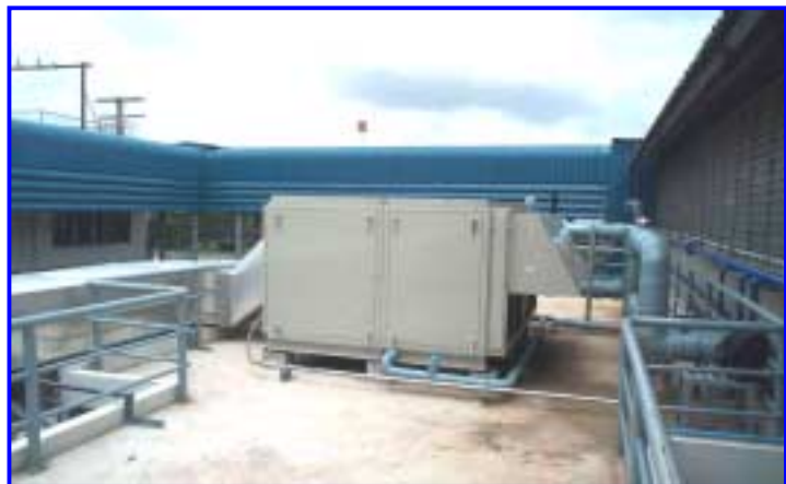
Fresh air unit has been used for better volume control and treat outdoor air to become neutral air.
