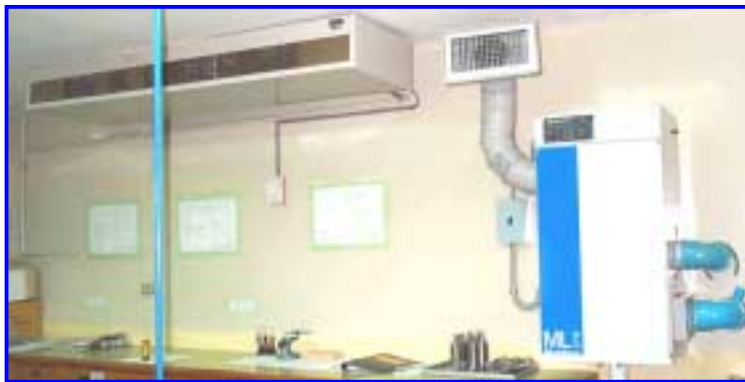
Standalone fresh air unit using desiccant wheel.
