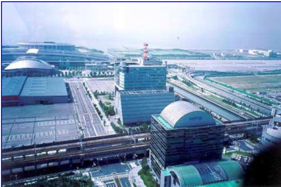
DHC Co-generation plant in Tokyo.
