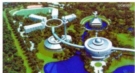
Shinawatt University uses District Cooling System.
