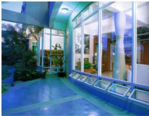
Example of ventilated window, which allows air intake at low level. This design is also very good to protect noise from neighbor. Shrub acts as air-filter.
