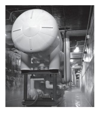
2. Stainless Steel Evaporative Condensers were used to withstand the tough ambient air and very high Hardness Water quality. However, water treatment and bleed off control are still essential to maintain the cooling water in good condition as much as possible.
