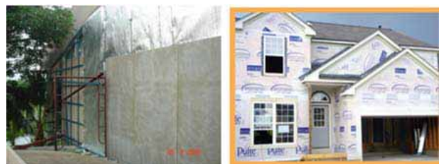
Figure 11. Installation of vapor barrier
