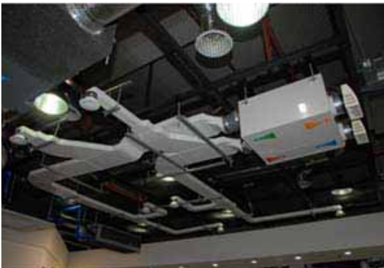
Figure 9. Fresh air unit with fresh air/exhaust air fan and air to air heat exchanger
