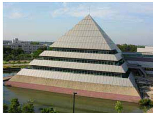
Figure 15. DEDE training center with low temperature air distribution system
