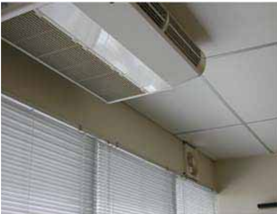
Figure 8. Installation of split type airconditioning unit with an exhaust fan
