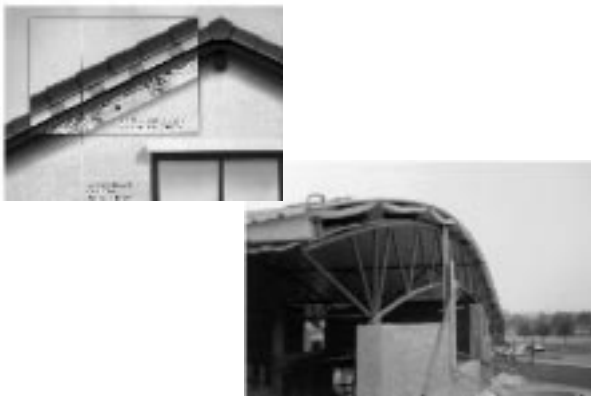
Insulation is the best method to protect heat. For example, when roof is well insulated, ceiling may not be further required to prevent heat.
