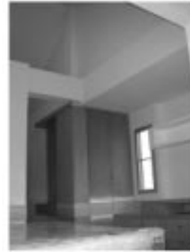
Upper floor of a town house with insulation and no ceiling.
