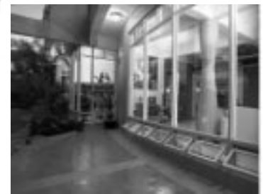
Example of ventilated window, which allows air intake at low level. This design is also very good to protect noise from neighbor. Shrub acts as air-filter.
