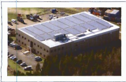
The rooftop solar array atop Ferreira's headquarters helps the building operate on net zero outside energy.
